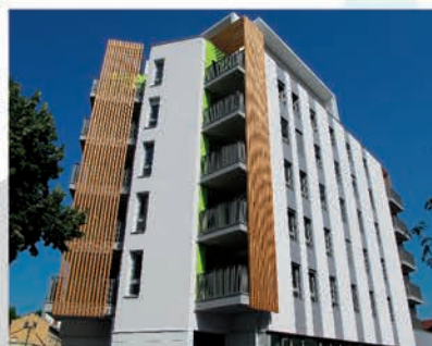
VILLEROY CREQUI - GRAND LYON HABITAT - Crèche 24 logements, LYON 3 ME
